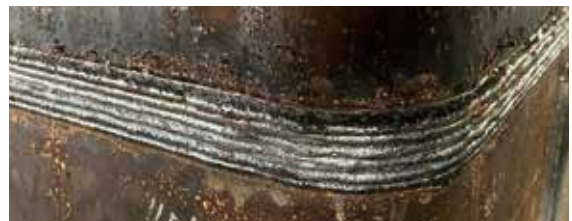
Column welding corner
