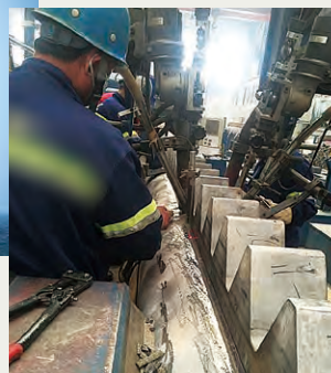
YP690 Rack & Chord 溶接風景 (SAW Y-80J x NB-250J)
