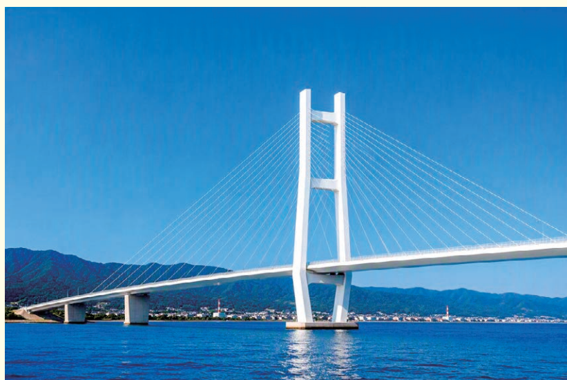
Kesennuma Bay Crossing Bridge
